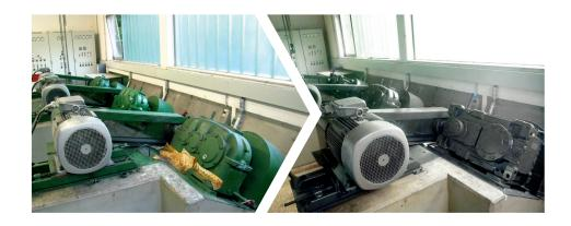
Left (before): **Drive variant B**Bevel-helical gear unit (third-party drive) with belt drive
