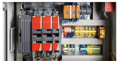
Compact control cabinet with MOVIDRIVE® modular
